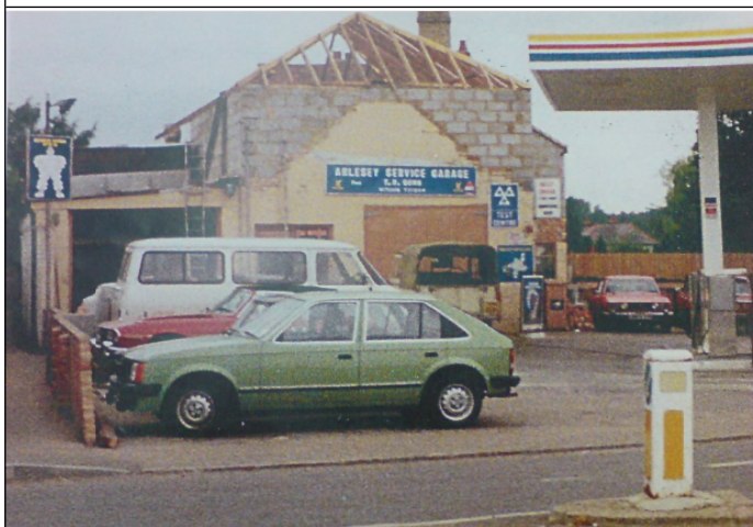
Photo taken in c.1970s Redevelopment to a two-story building with two work bays. The apex of the original building is marked by the rendered surface.
